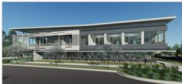
Florida Public Utilities Office
