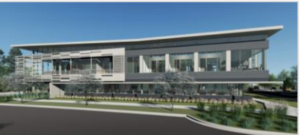
Florida Public Utilities Office
